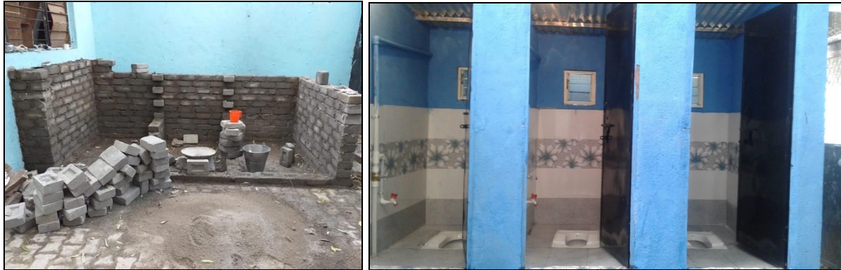
Toilet Construction completed at Synergy Pune Home
