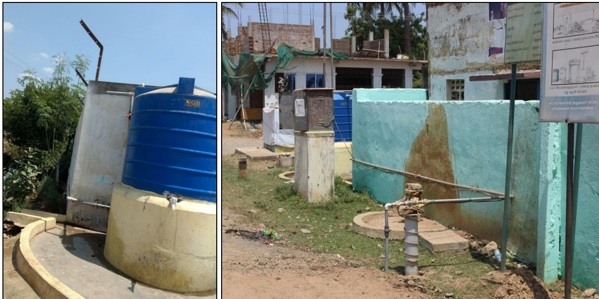
Water Supply Connections at Chithukadu Panchayat
